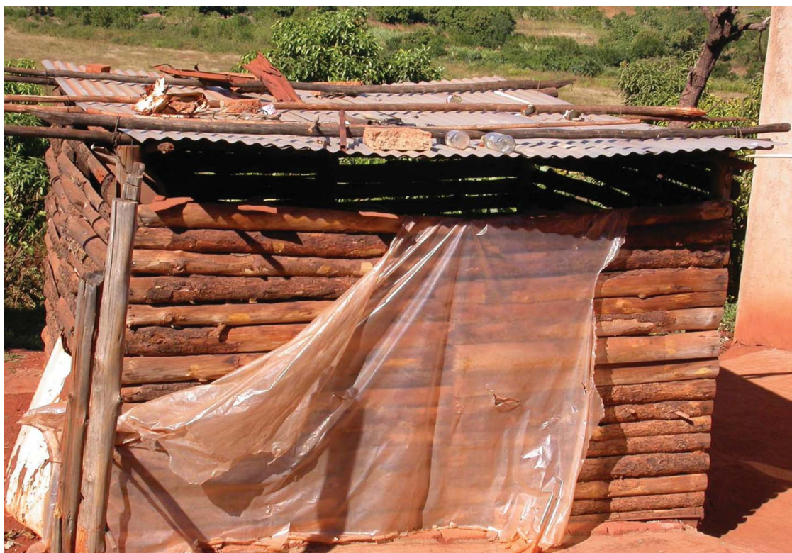
Figure 1 An inappropriate store in rural area of Limpopo province of South Africa, which would not be able to preserve feed from rain. (Color figure available online.)
