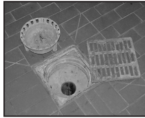
Figure 8. Floor drain and dairy brick flooring surface.
