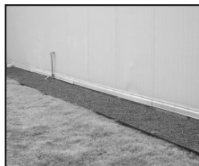
Figure 7. Pebble rock strip around production facility.
