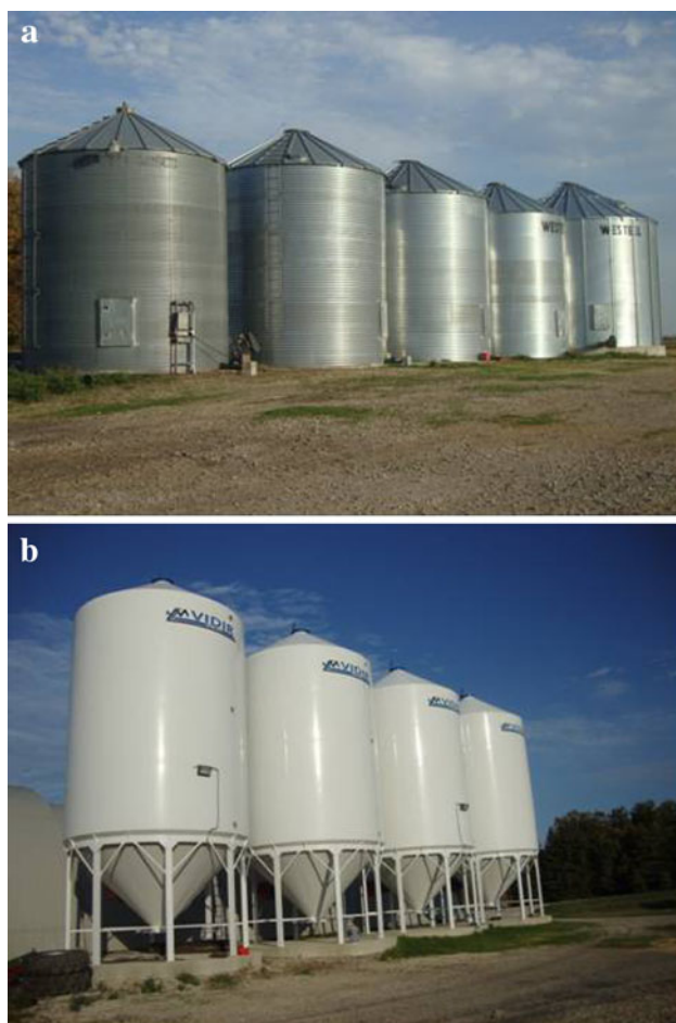
Fig. 1 a An example of good storage system using flat-bottom bins with aeration and drying capabilities. b An example of good storage system using hopper-bottom bins with aeration and drying capabilities
