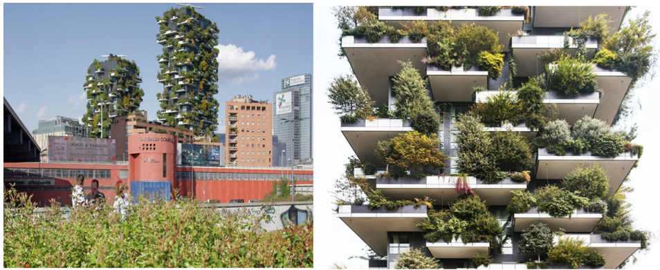
Fig. 5 The Vertical Forest suburb El Bosco in Milan with 27-storey apartment buildings with planted balconies. Source Vertical Forest (2018)
