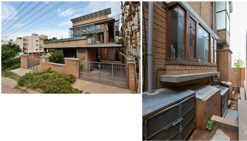
Fig. 6 The ecohouse with solar panels and gated gardens (left), and the treatment units at the back of the house (right). Source Ecohouse (2014)
